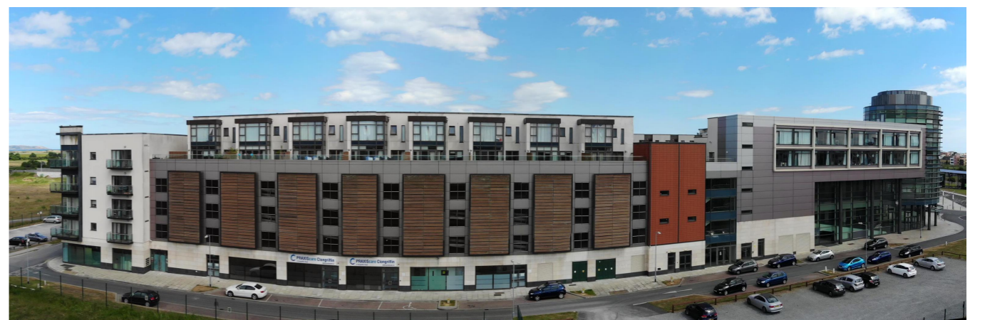
Block 12 was completed in 2008
