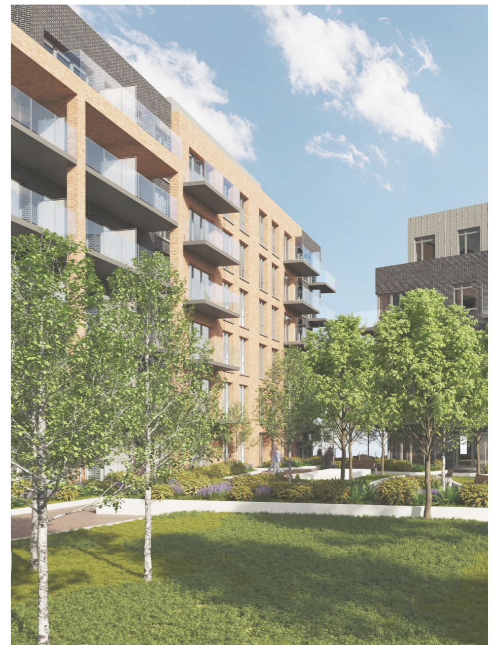
View of Block 8 podium level landscaped courtyard
